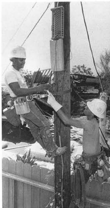
Left. A Southwestern Bell lineman takes down a storm-damaged cable.
